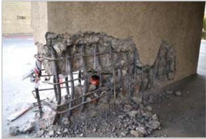
Fig.1 Flexure failure through concrete crushing
