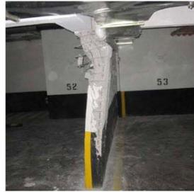
Fig.2 Out-of-plane buckling failure
